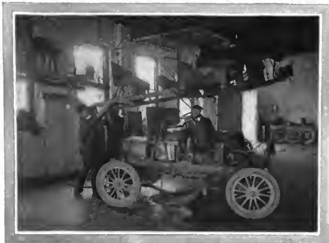
LOWERING TESTING BODY ON THE CHASSIS.
